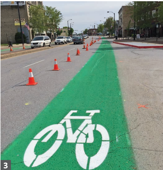
1 Use push brooms to remove debris from the street. Measure at least 6 feet from the curb, mark with chalk spray, then mark every 15 feet along the lane and use a snap chalk line to connect the marks. Duct tape can be used along this line to define the edge while painting.
