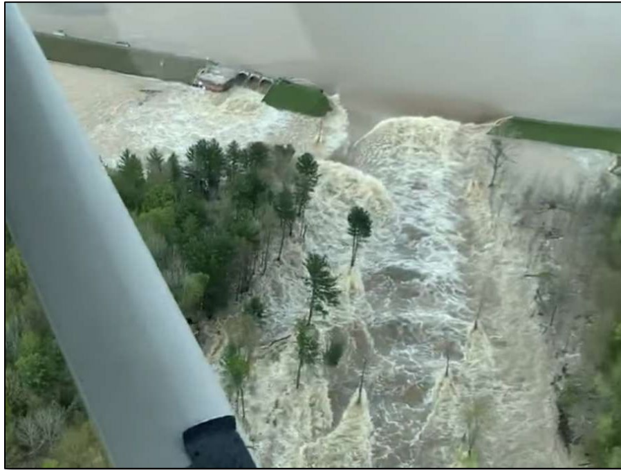
Figure 47: Ariel Footage of Edenville Dam Failure
