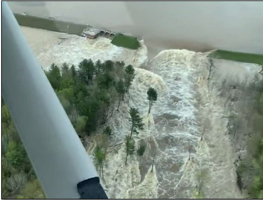
Figure 52: Ariel Footage of Edenville Dam Failure
