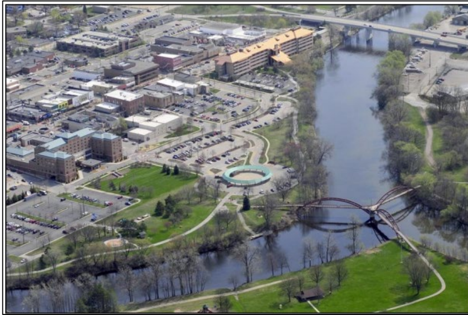
Figure 54: Before Flooding Depiction Beside the Tittabawassee River
